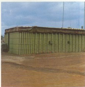
Typical Battery FDC
