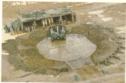
8"/175 Gun Pad with retaining wall
